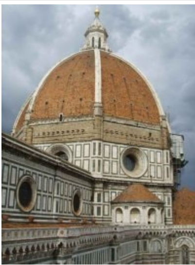
Dome of the Florence Cathedral, designed by Filippo Brunelleschi (Creative Commons [3] )
